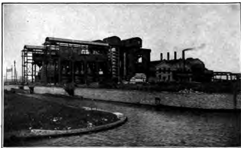
FIG. 252.—Mond Byproduct Gas Plant, at Dudley Port, South Staffordshire, England.
